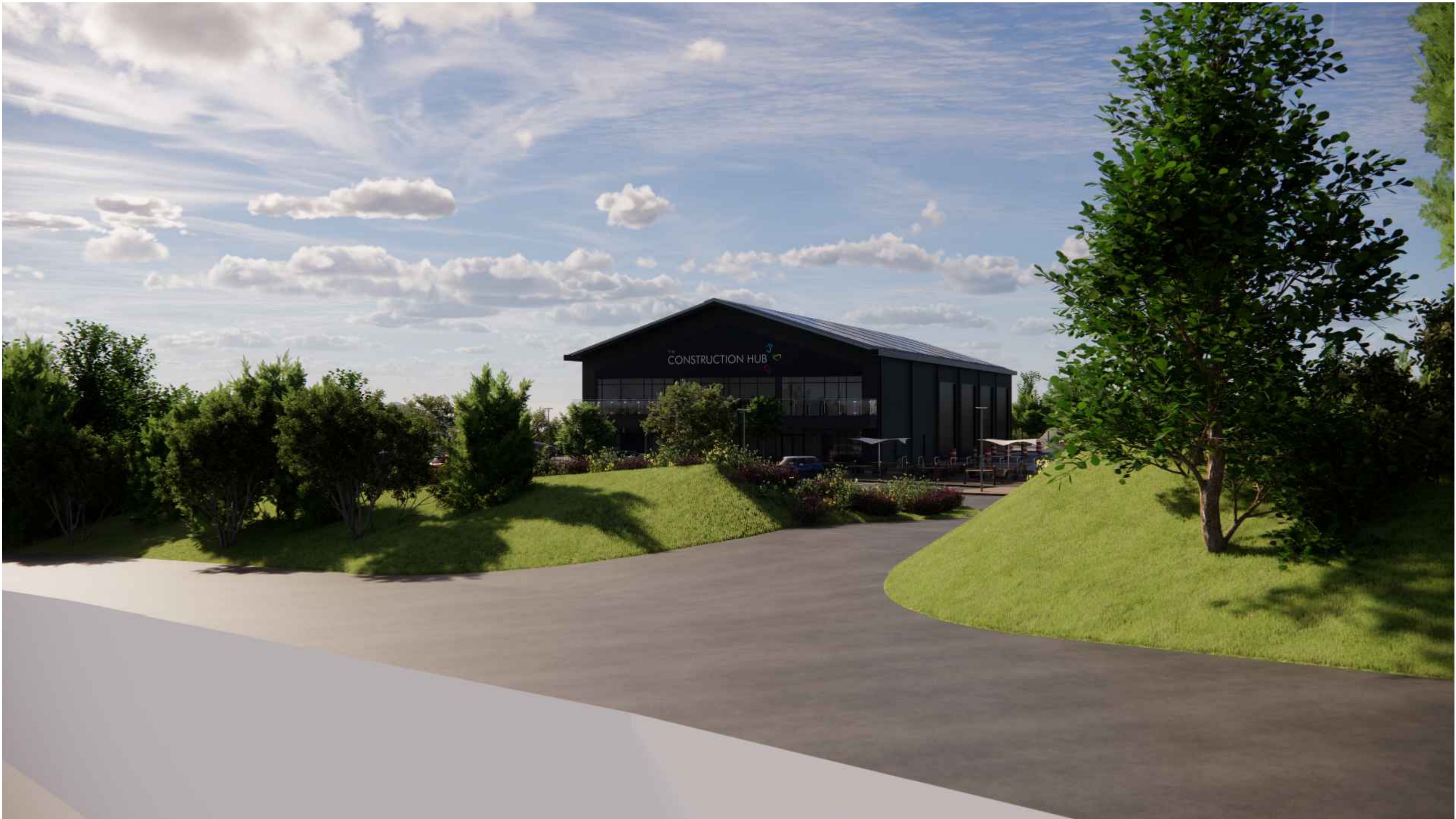
Southbound View Along Parkway of Proposed Site Access Junction, Showing Proposed Construction Hub in Background
