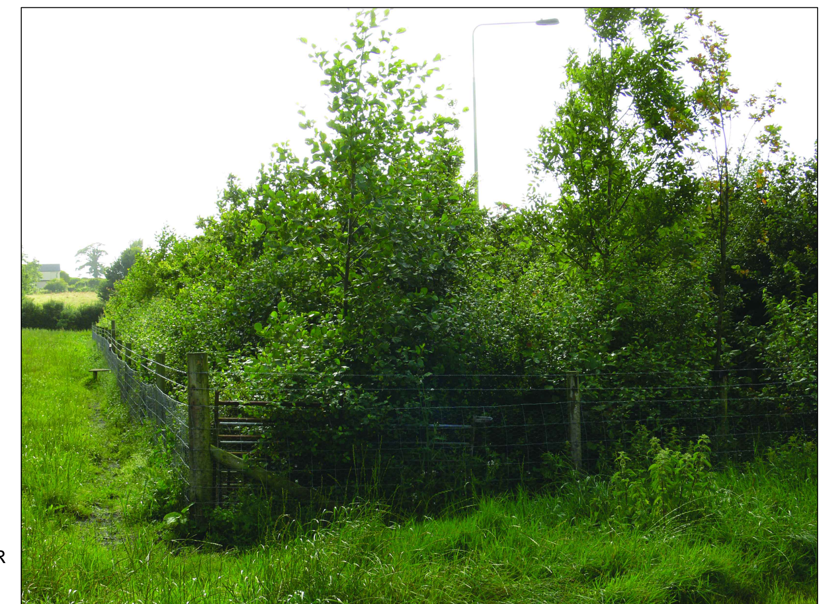
SITE AT INSPECTION, 4 MONTHS AFTER PRACTICAL COMPLETION
